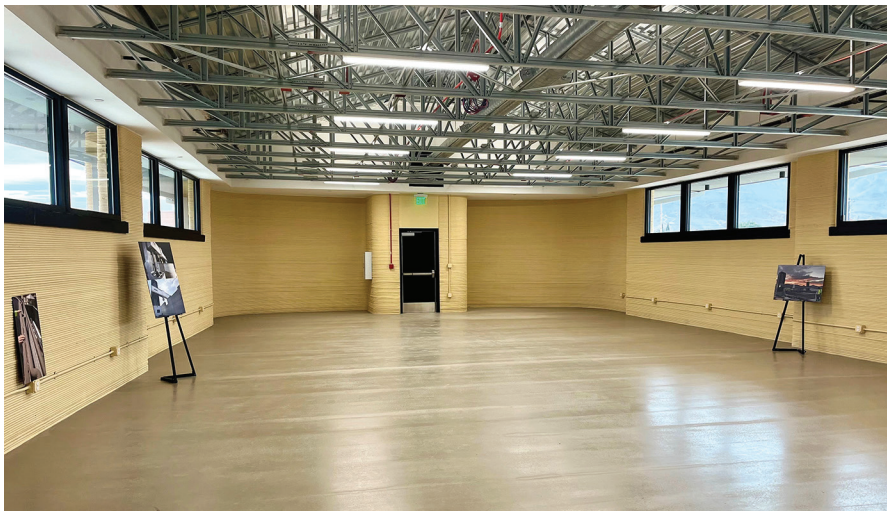
The 3D-printed facilities will be used as collective training barracks, each featuring 36 bunk beds that can house up to 72 soldiers. (U.S. ARMY/ALYX RIEBELING)
