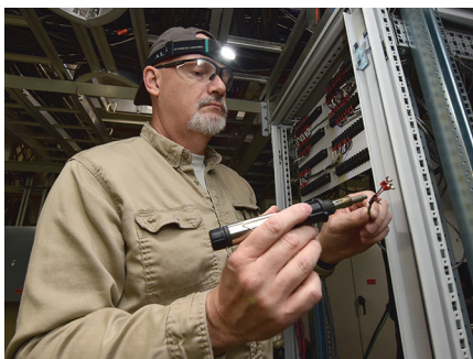
Journeyman electrician Waylon Hackett, of the Army Corps of Engineers Nashville District, solders wiring analog inputs during installation of a supervisory control and data acquisition system at the Dale Hollow Dam Power Plant in Celina, Tennessee. (U.S. ARMY/LEON ROBERTS)
